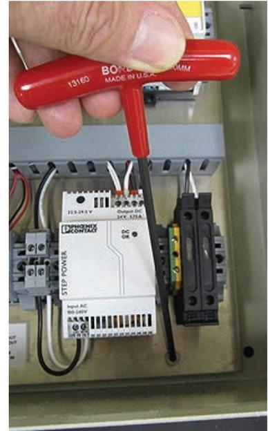
Back plane assembly securing bolt locations
