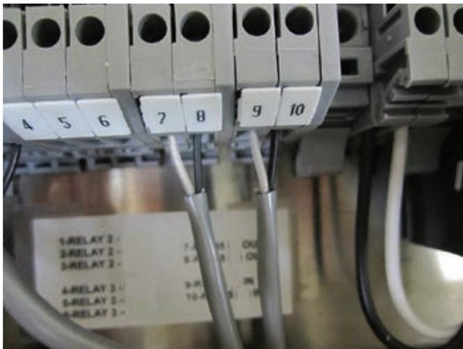
5. Connecting sensor circuit leader cables to internal SIMs.
